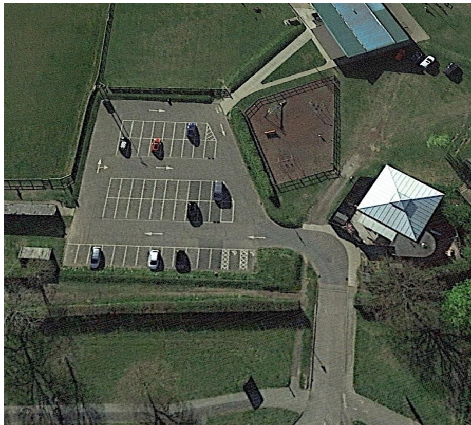
figure 50: The Existing Chilton Fields Car Park
