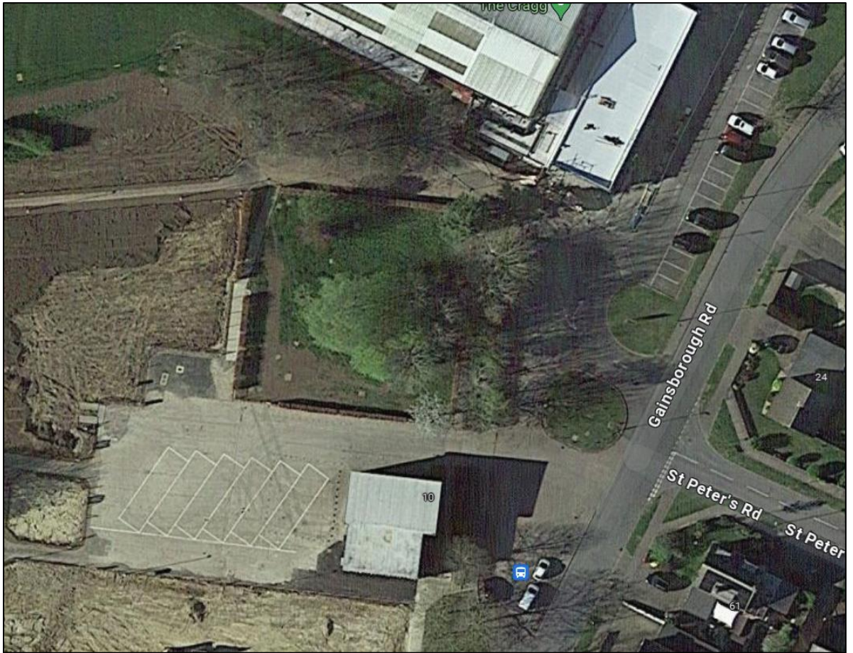
figure 71: Existing Vehicular Access point Gainsborough Road
